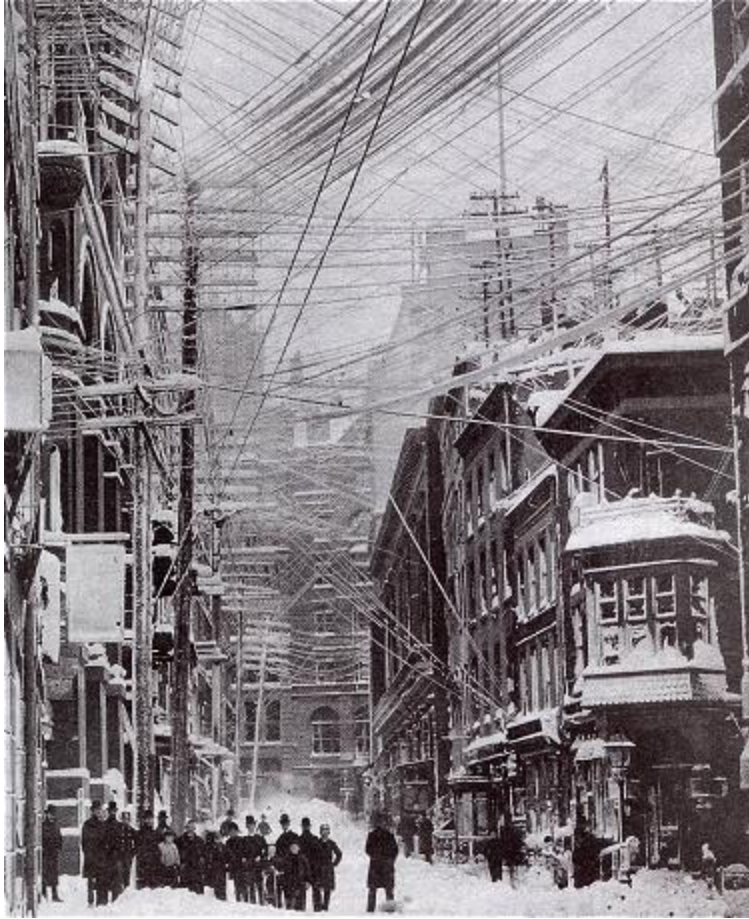
Figure 4 Chaos of Telephone, Telegram, and Power lines NYC 1880 before monopolies were granted. Credit: Wikipedia 11
